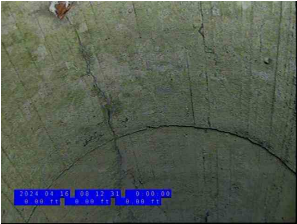
5, 00:00:52, 0.00ft Crack Multiple from 12 o'clock to 12 o'clock, Start
