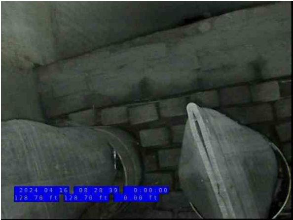
14, 00:14:09, 130.00ft Obstruction Brick or Masonry, 55% of cross sectional area from 3 o'clock to 9 o'clock
