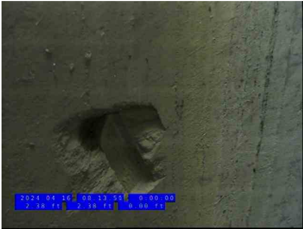
6, 00:01:38, 2.38ft Surface Damage Missing Wall at 10 o'clock
