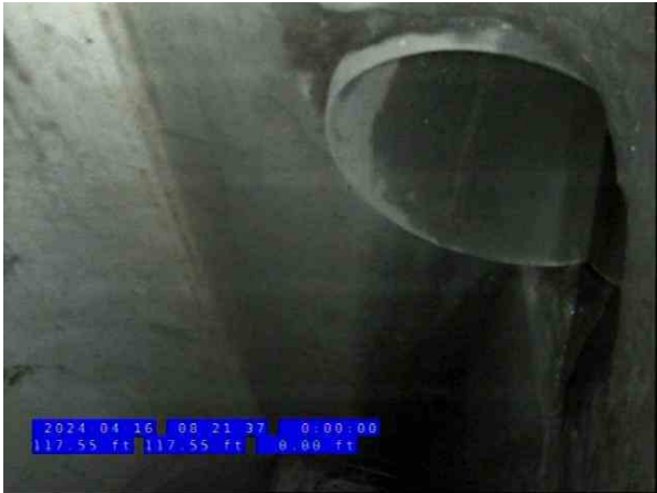
8, 00:08:03, 117.55ft Tap Break-in/Hammer at 4 o'clock, dia/height: 15inch / 12-15
