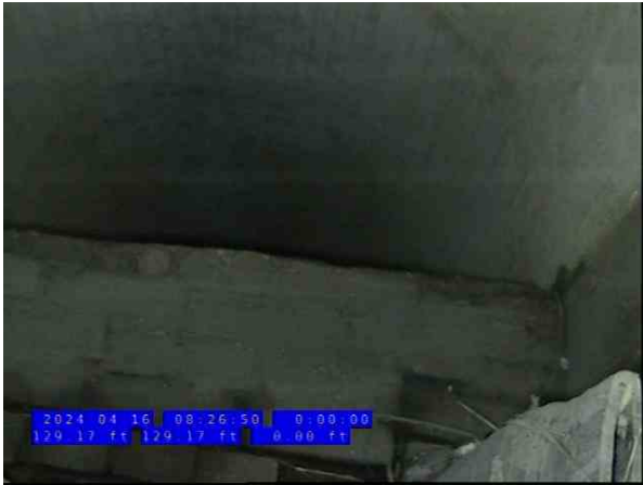
10, 00:13:07, 129.00ft Deposits Settled Fine, 5% of cross sectional area from 4 o'clock to 8 o'clock, Finish
