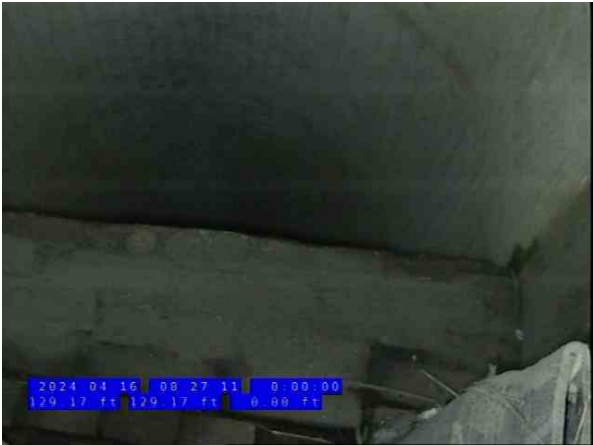
11, 00:13:11, 129.00ft Crack Multiple from 12 o'clock to 12 o'clock, Finish
