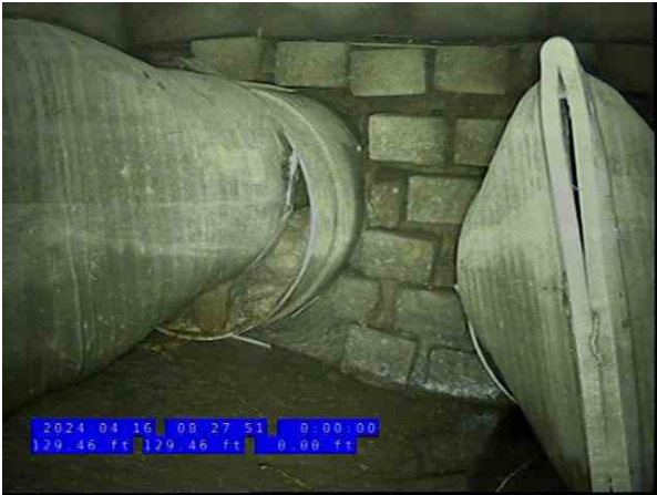
13, 00:13:23, 129.00ft Miscellaneous General Observation / SEPERATION
