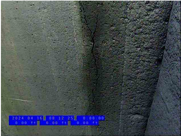
4, 00:00:52, 0.00ft Crack Multiple from 12 o'clock to 12 o'clock, Start
