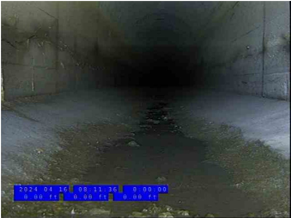
3, 00:00:12, 0.00ft Deposits Settled Fine, 5% of cross sectional area from 4 o'clock to 8 o'clock, Start
