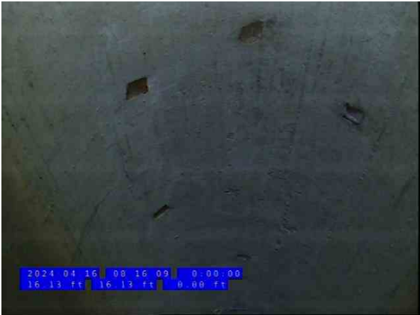
7, 00:03:35, 16.13ft Miscellaneous General Observation / POSSIBLE HOLE. COULD BE FOR GROUND WATER
