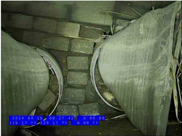
12, 00:13:23, 129.00ft Miscellaneous General Observation / SEPERATION
