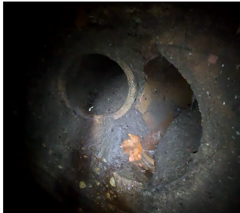
only pipes visible in overflow chamber. on wall adjacent to tide gate
