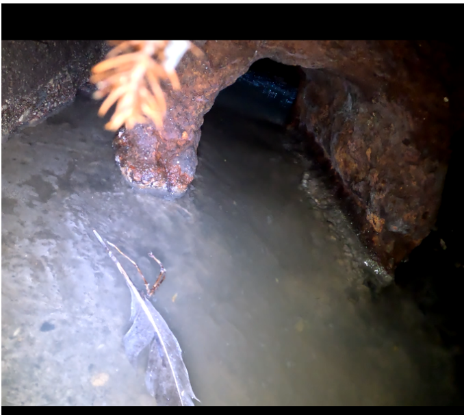
opening between regulator and inlet chambers
